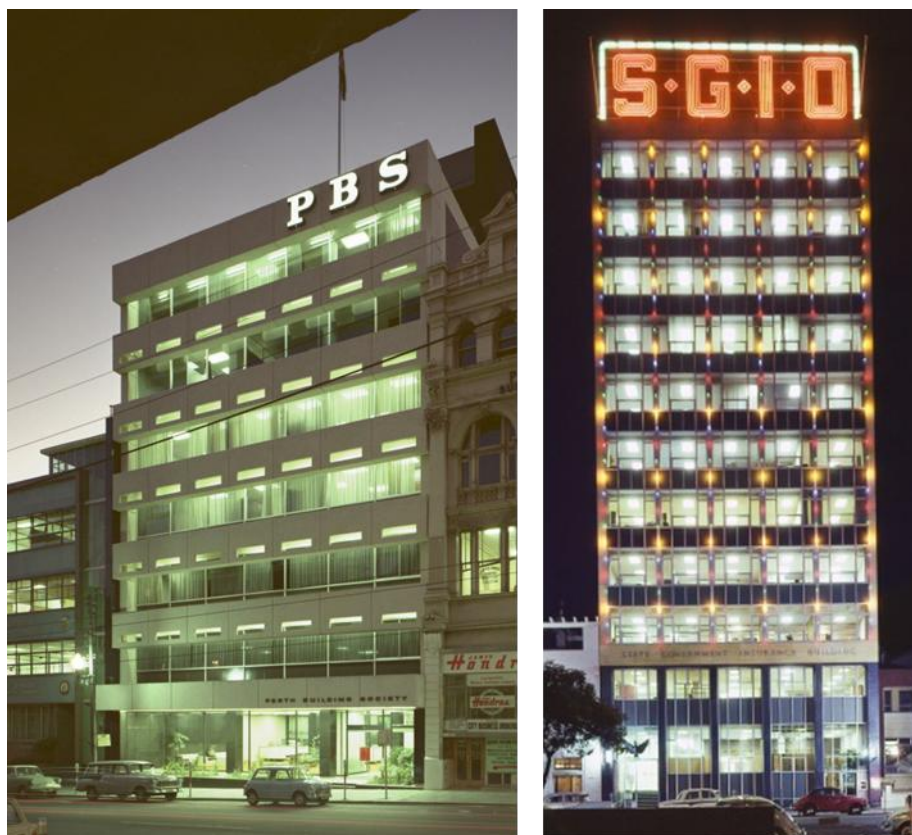
Figure 14: The new PBS and SGIO buildings
